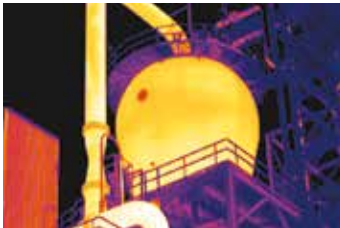
Refractory insulation inspection on a petrochemical reactor
