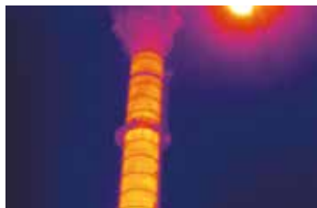
Refractory material inspection on a furnace chimney.
